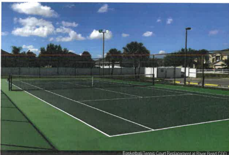
Basketball/Tennis Court Replacement at River Bend CDD
