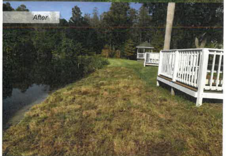
Pond Restoration at Westchase CDD
