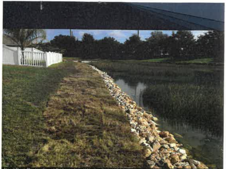
Pond Bank Restoration at Bridgewater of Wesley Chapel CDD
