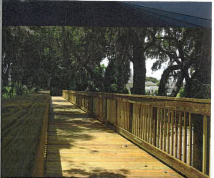
Pedestrian Boardwalk at Oak Creek CDD
