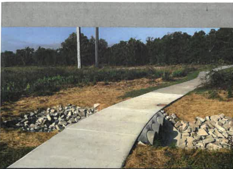
Sidewalk Repairs at Fishhawk Ranch CDD
