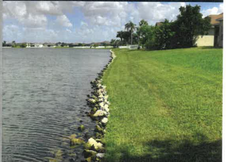
Pond Bank Restoration at Mira Lago CDD
