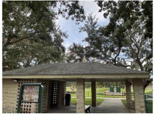
Asphalt shingle overview with discoloration at shingles and fascia board
