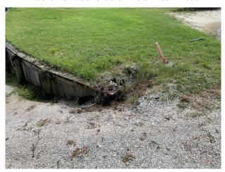
Erosion at end of Hole 7 bulkhead
