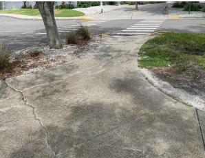
Concrete sidewalk with cracks and trip hazards at Clubhouse
