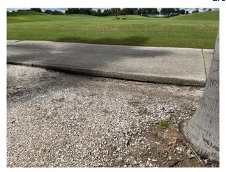
Soil undermining cart path at graveled area
