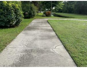
Concrete sidewalk with cracks and settlement near Fawn Ridge
