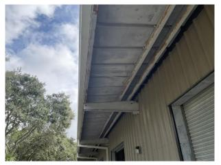
Structural steel frame with rust evident
