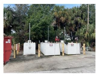
Gasoline, diesel fuel and oil separation storage tanks
