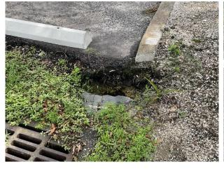
Soil undermining pavement at drainage area
