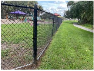
Chain link fence at dog park with warped webbing
