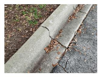
Concrete crack with tree root upheaval at Woodside Park
