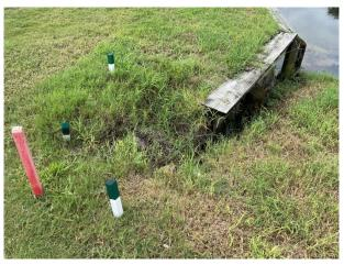
Erosion at end of Hole 7 bulkhead
