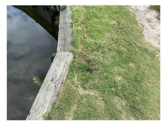
Erosion at backside of Hole 7 bulkhead
