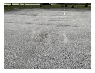
Pavement cracks and settlement
