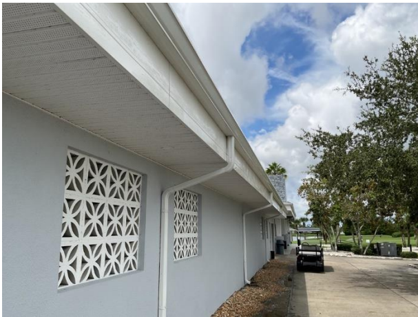
Aluminum gutters and downspouts
