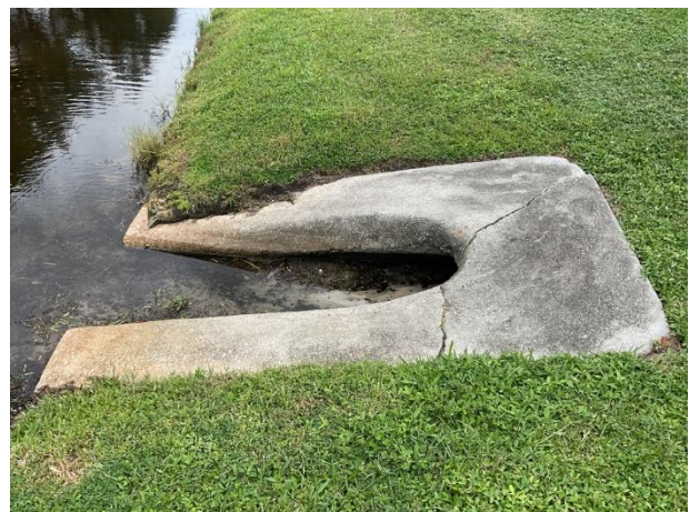
Pond inlet structure
