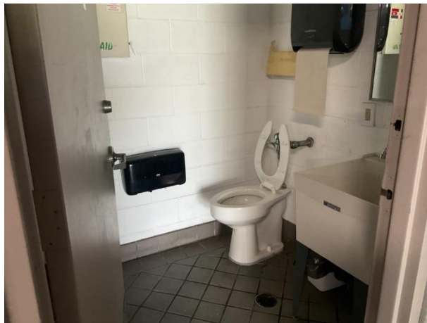
Rest room at cart barn
