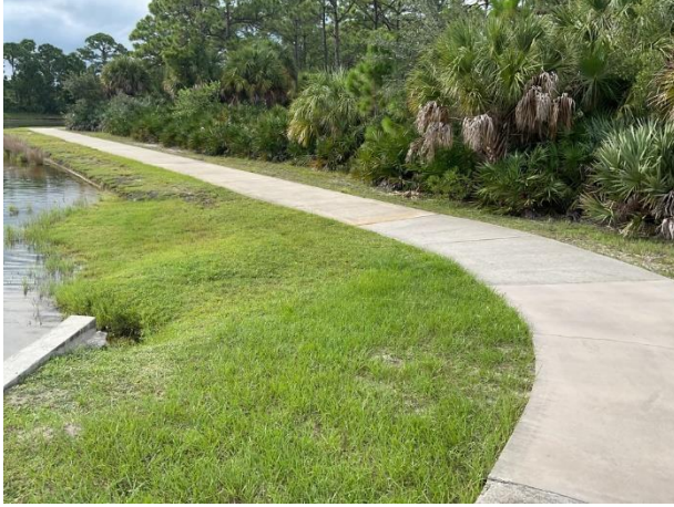
Concrete sidewalk overview on island
