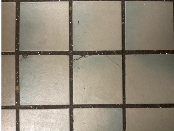
Tile cracks
