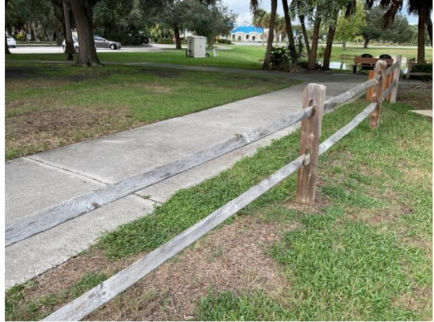
Wood split rail fence at playground area
