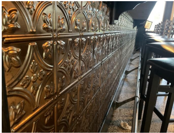
Plastic covering at bar
