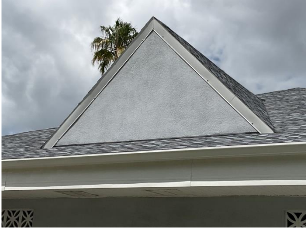
Stucco terminates above lower roof section
