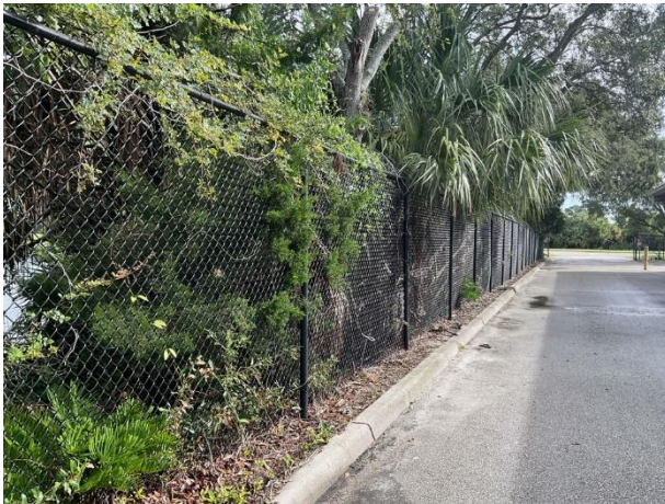
Chain link perimeter fence at maintenance facility
