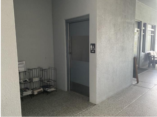
Metal door at rest room
