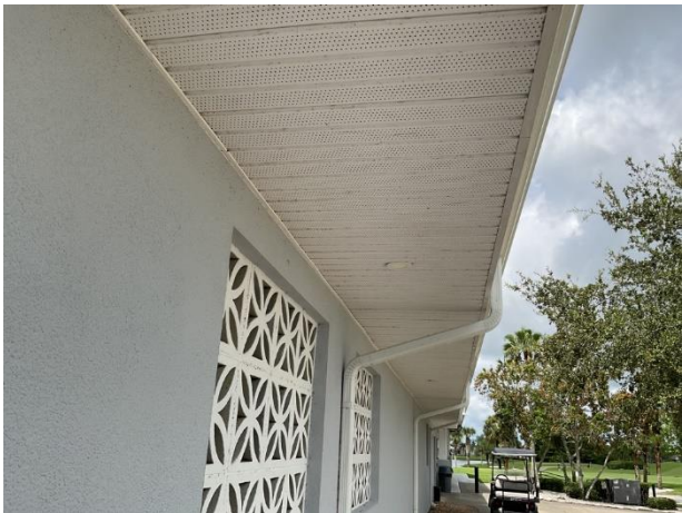
Vinyl soffits and fascia at Clubhouse
