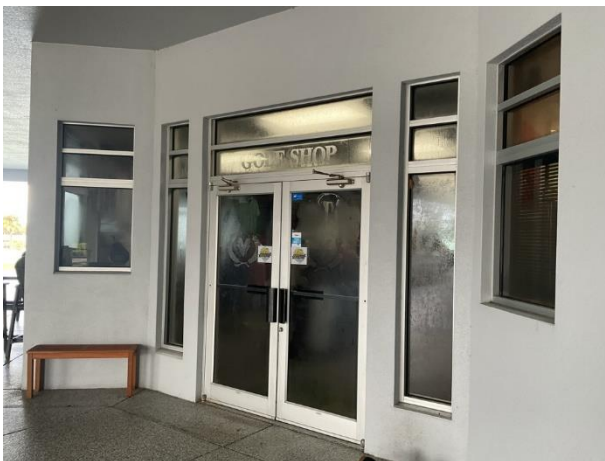
Windows and doors at Pro Shop
