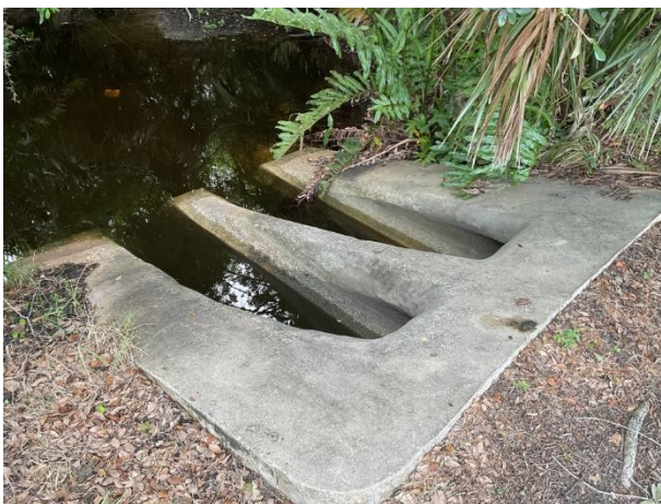
Overflow outlet structure
