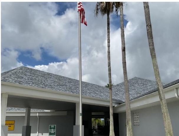
Roof overview at portico
