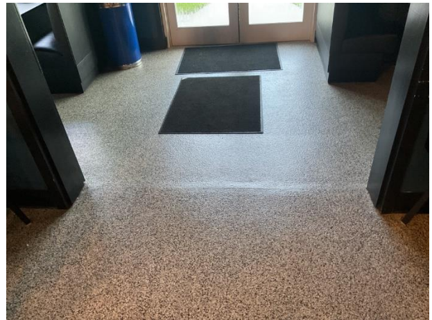
Gemstone floor coating inside restaurant
