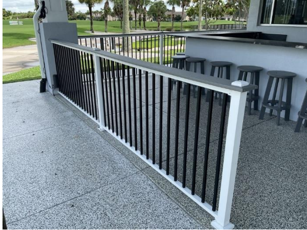
Aluminum railings at outdoor seating area
