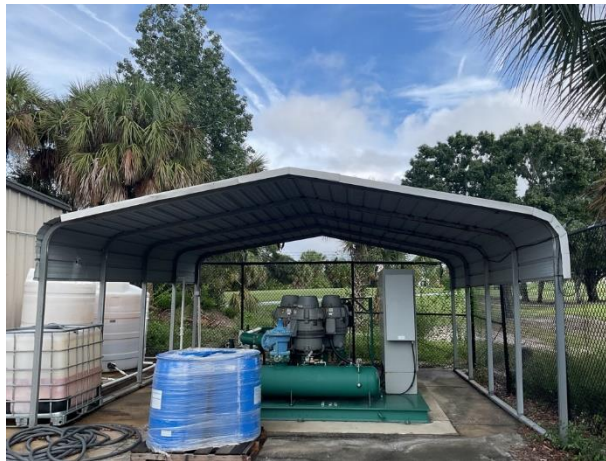
Carport at irrigation system pump station
