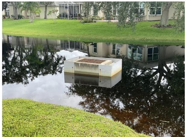
Pond control structure
