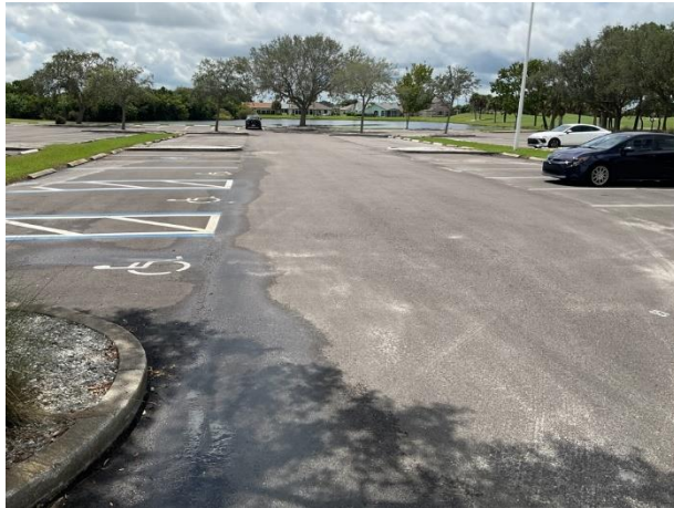
Pavement parking area overview at the Clubhouse
