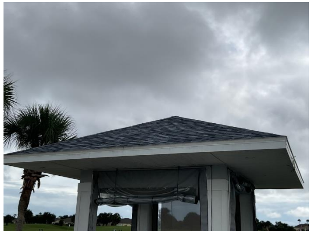
Roof at Starter's Station
