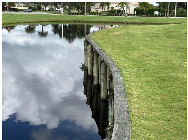
Timber bulkhead overview
