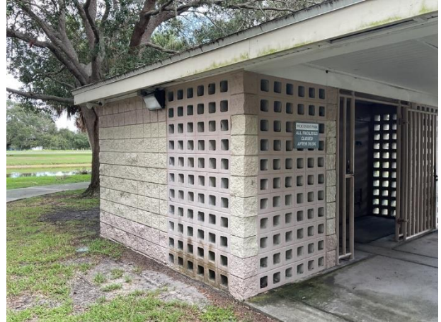
Paint finishes at concrete façade
