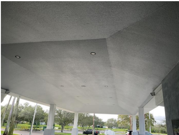
Stucco finishes at portico
