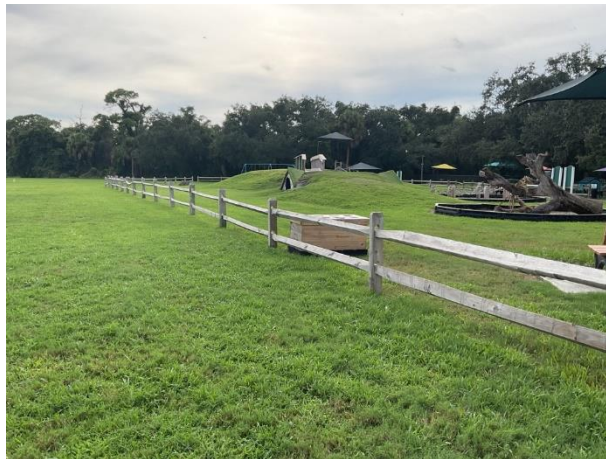
Wood split rail fence at playground
