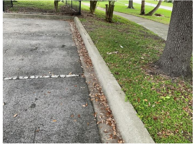
Concrete curb and gutter at Woodside Park
