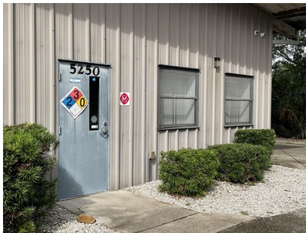
Windows and doors at maintenance office
