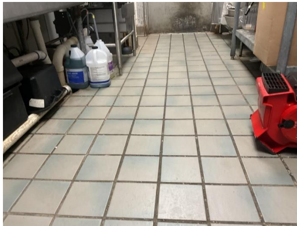
Tile floor coverings at dishwashing area
