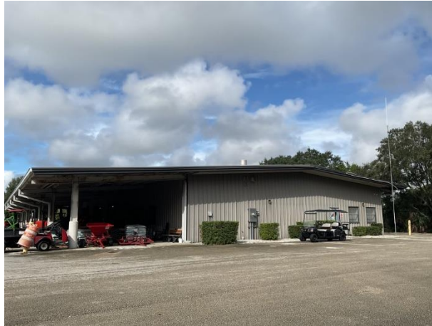
Maintenance building exterior overview
