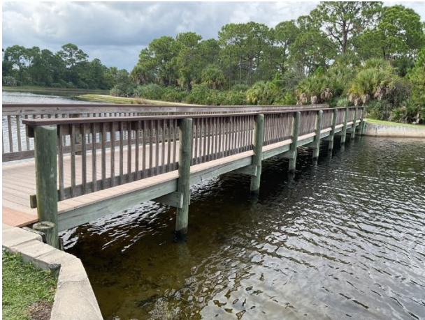
Bridge with wood structure and railings and composite deck boards
