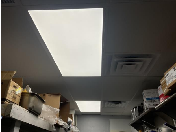
Acoustical ceiling at kitchen
