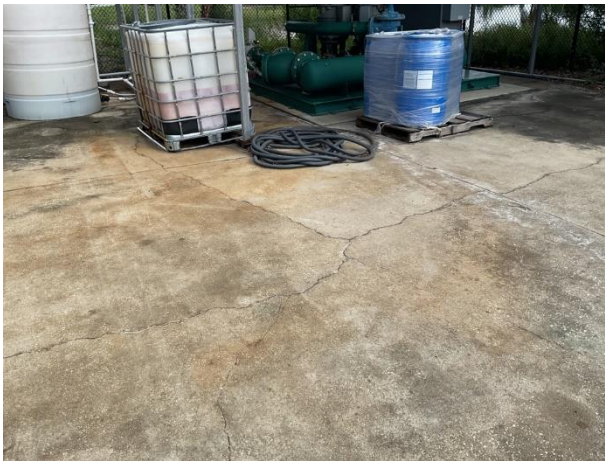
Concrete flatwork near pump station
