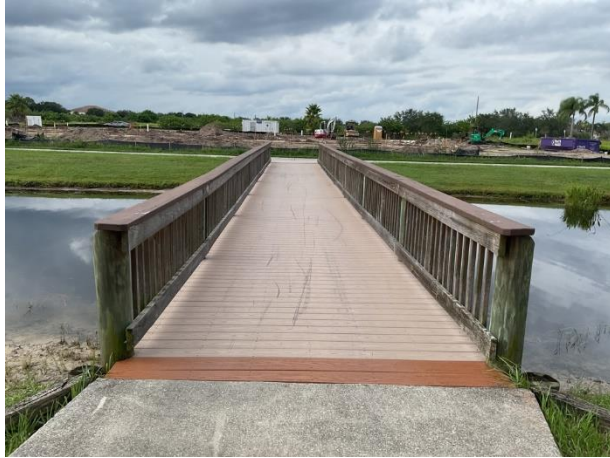
North bridge overview
