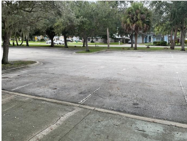
Asphalt pavement parking area overview at Woodside Park
