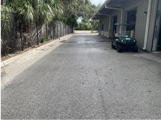
Asphalt pavement at maintenance facility
