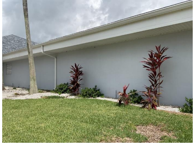
Stucco wall finishes at cart barn
