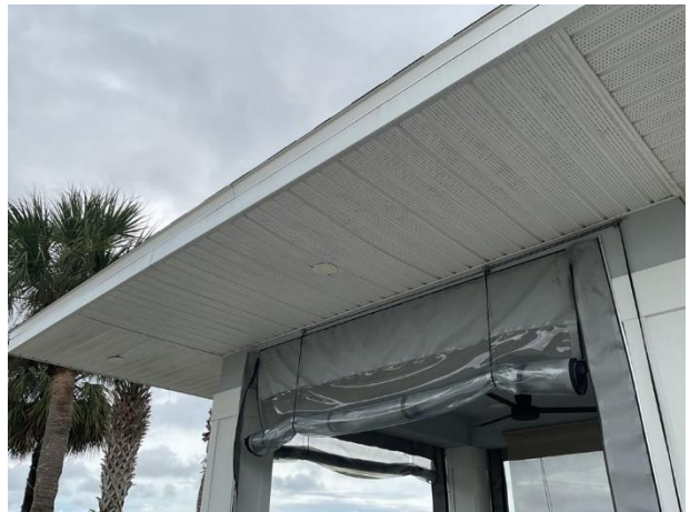
Vinyl soffits and fascia at the Starter's Station
