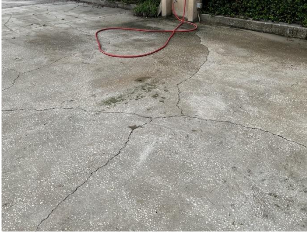
Concrete cracks
