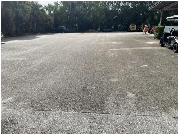
Pavement parking area overview
