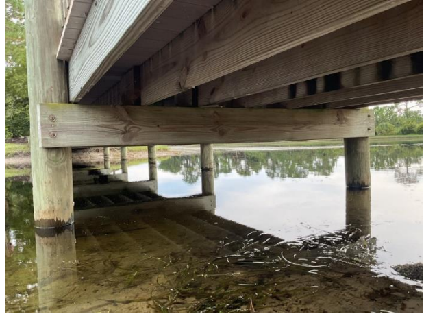
Bridge structure overview
