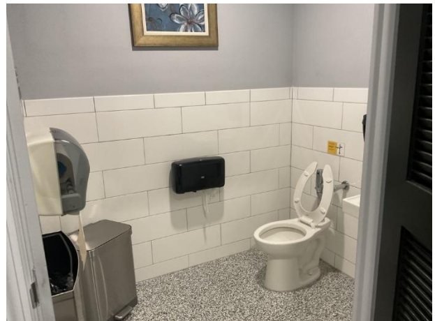
Rest room fixtures and finishes
