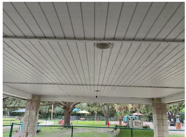
Wood ceiling at patio
