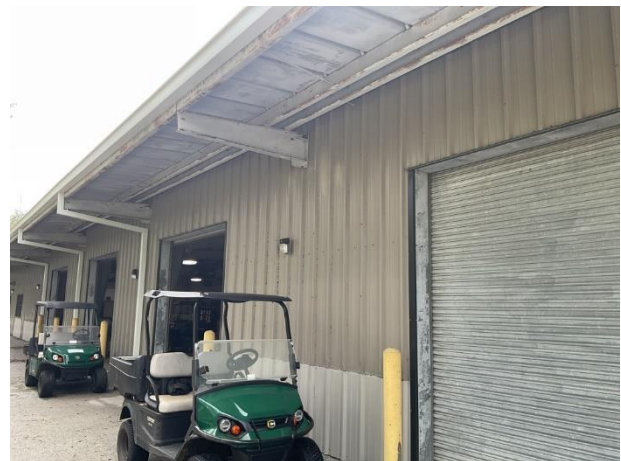
Metal siding at maintenance building
