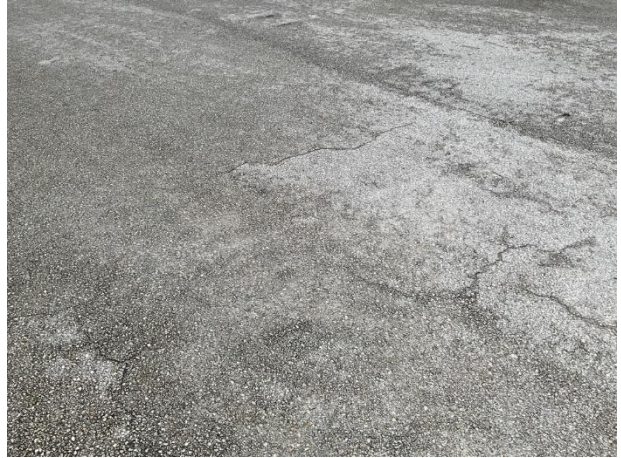
Pavement cracks
