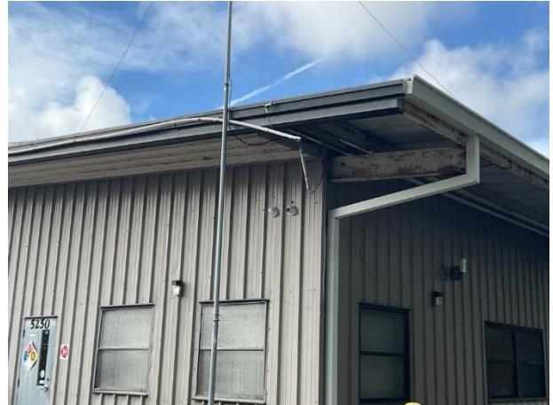
Security system cameras at maintenance facility
