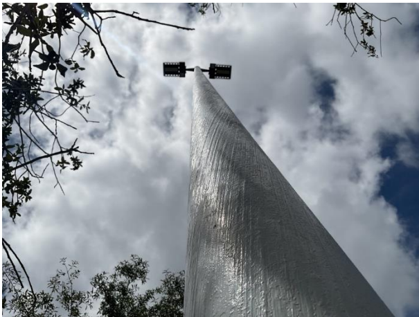
Fiberglass light pole with paint finishes
