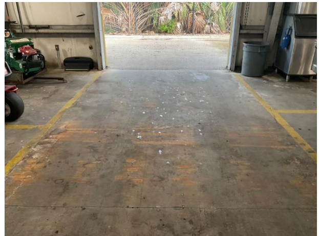
Concrete parking surface at maintenance building
