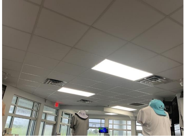
Acoustical ceiling at pro shop
